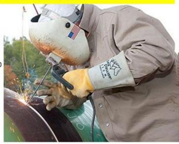
Pipe welding is a demanding field, where every weld must meet the most stringent construction codes in the industry. Piping systems are the backbone of any major factory or plant, transporting fluids for power or processing needs. These systems can carry high-temperature or high-pressure materials and must be built with the highest standards of quality and safety in order to protect the workers and the community they serve. As a pipe welder, you are responsible for every weld you make.
